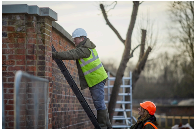
Putting in the wires in the walled garden
